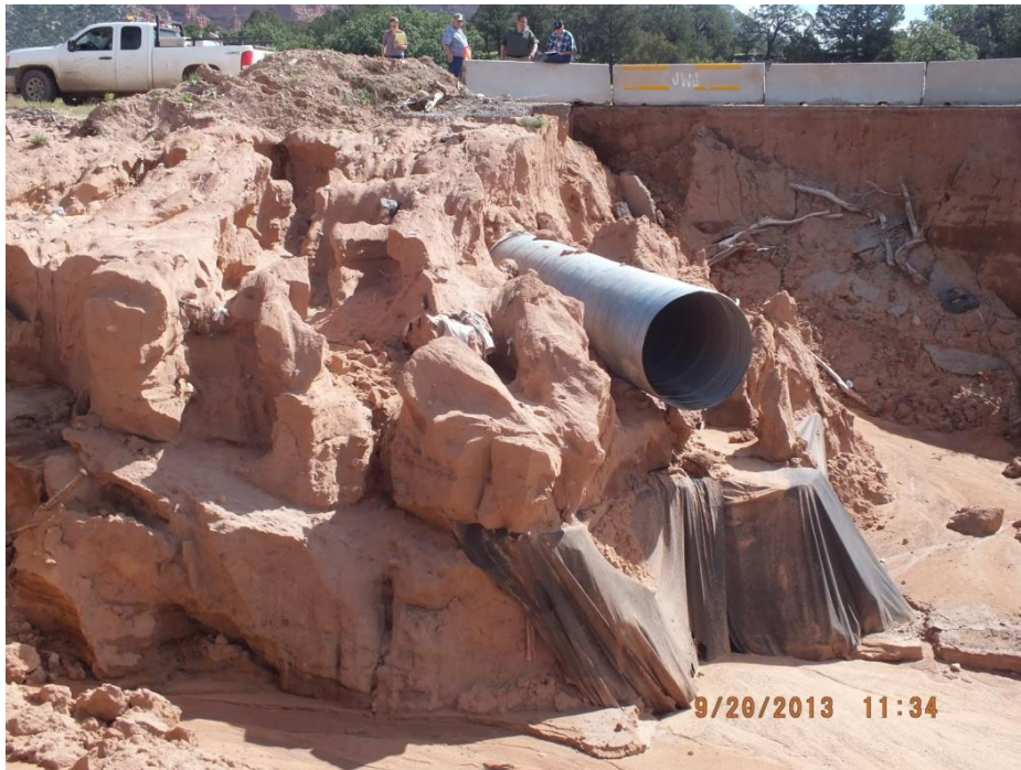
Figure 19: State Route 61 Washed Out by Flash Flooding
