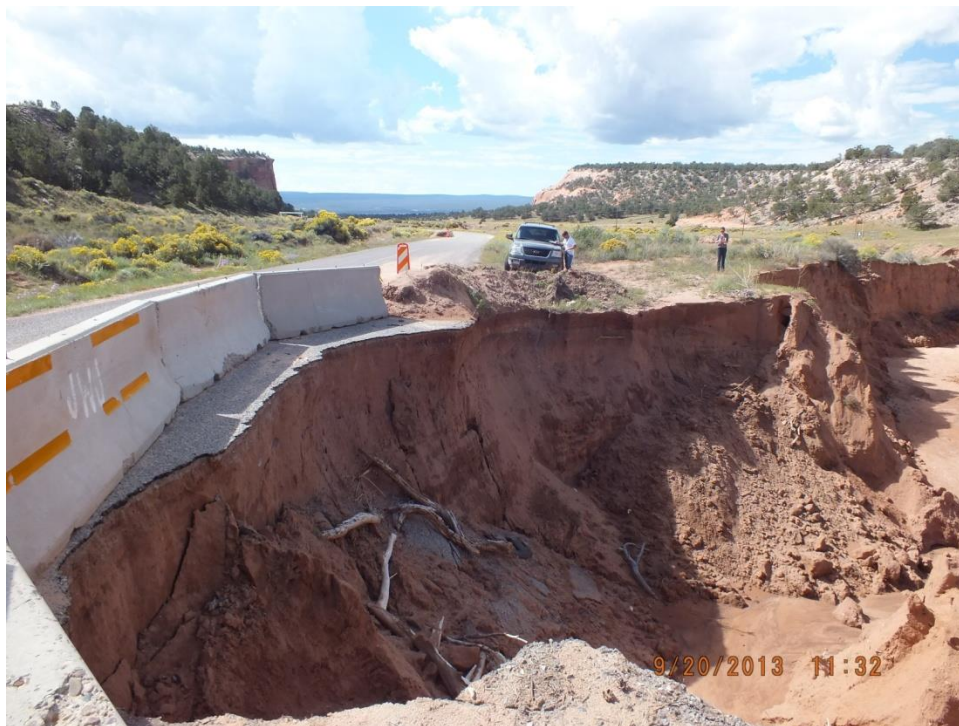
Figure 20: State Route 61 Washed Out by Flash Flooding
