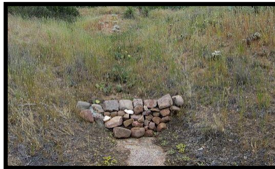
Image 3 a check dam stabilizes soil behind it
